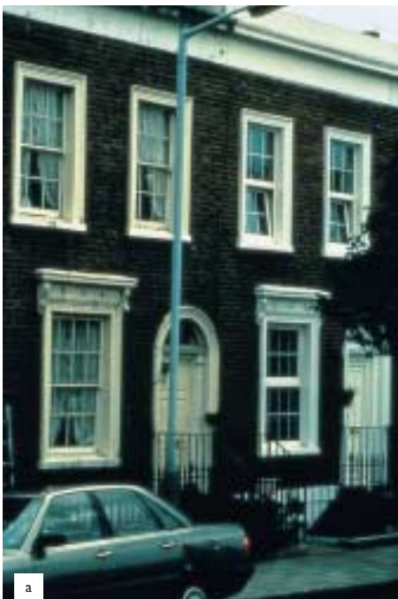
Figure 1 (a, above) Double glazing in PVCu cannot replicate the appearance of an original timber sash with fine glazing bars. (b, right) An unfortunate combination on the same façade: original timber sashes (ground floor), PVCu replacements (first floor) (Photographs: Chris Wood and English Heritage Building Conservation and Research Team)
