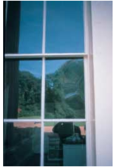
Figure 5 Historic glass, especially Crown glass, is rare and cannot be reproduced today. Where examples such as the middle right pane survive, they must be preserved. (Photograph courtesy of Treve Rosoman)
